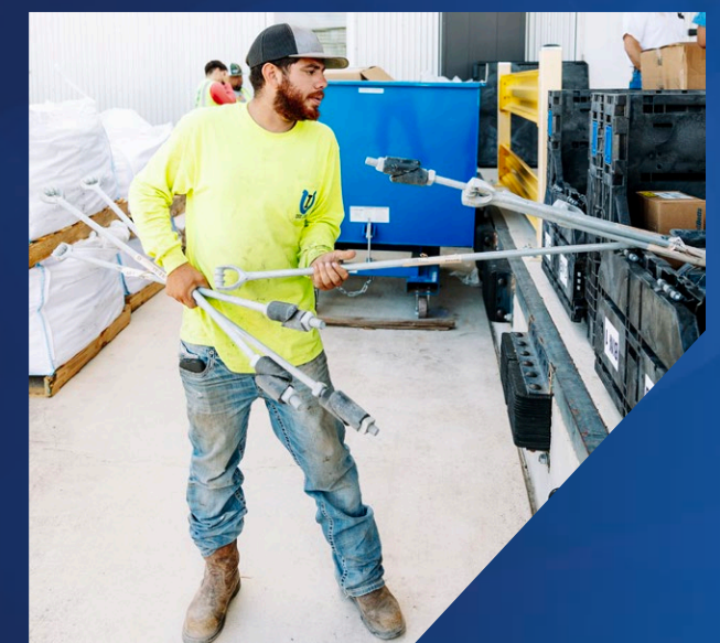
Construction crews unload a pallet of much needed rock anchors for the next fiber project on their list.
